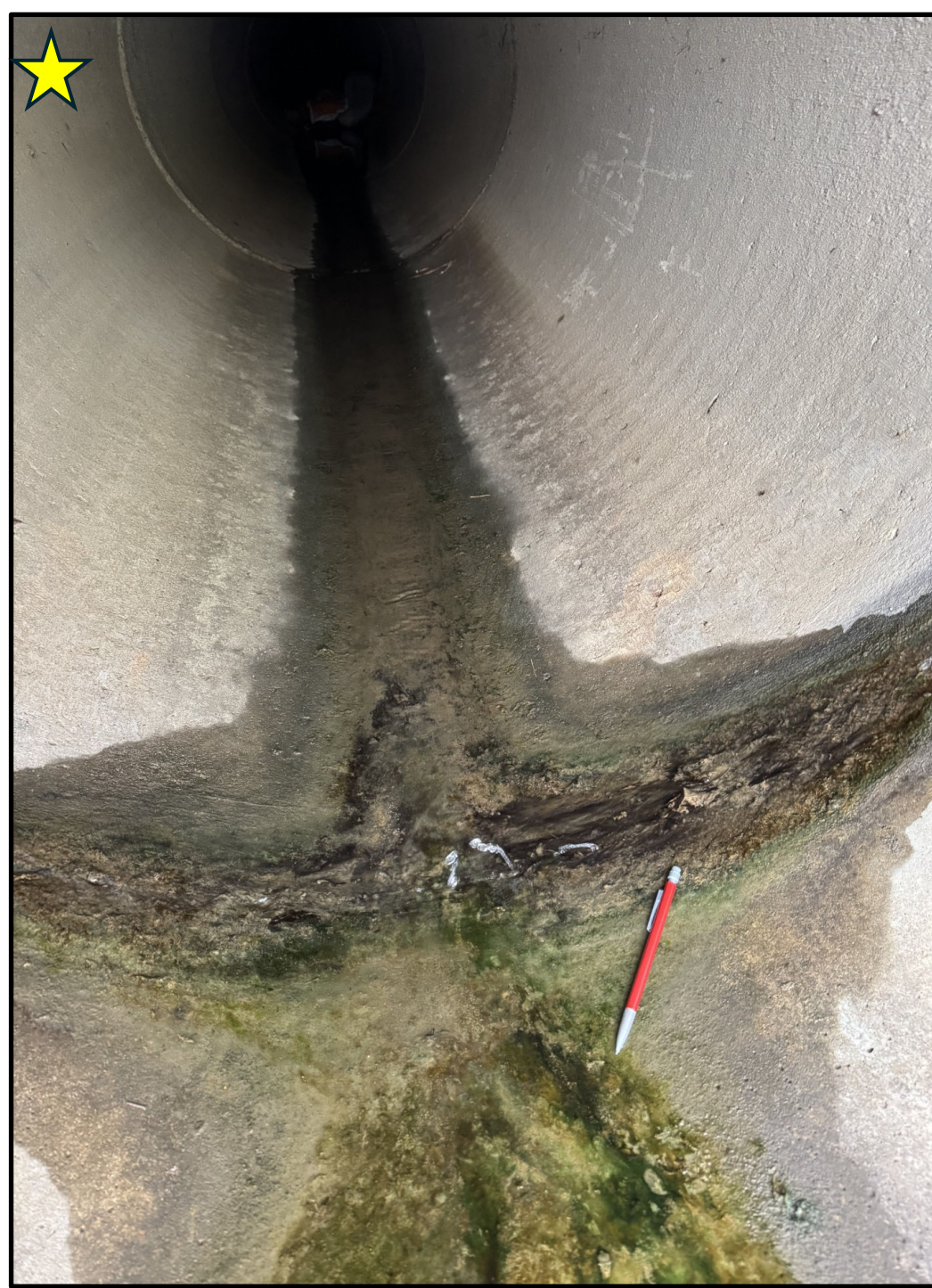
Figure 7: Artesian flow at the entrance of the main culvert that flows to site 3.
