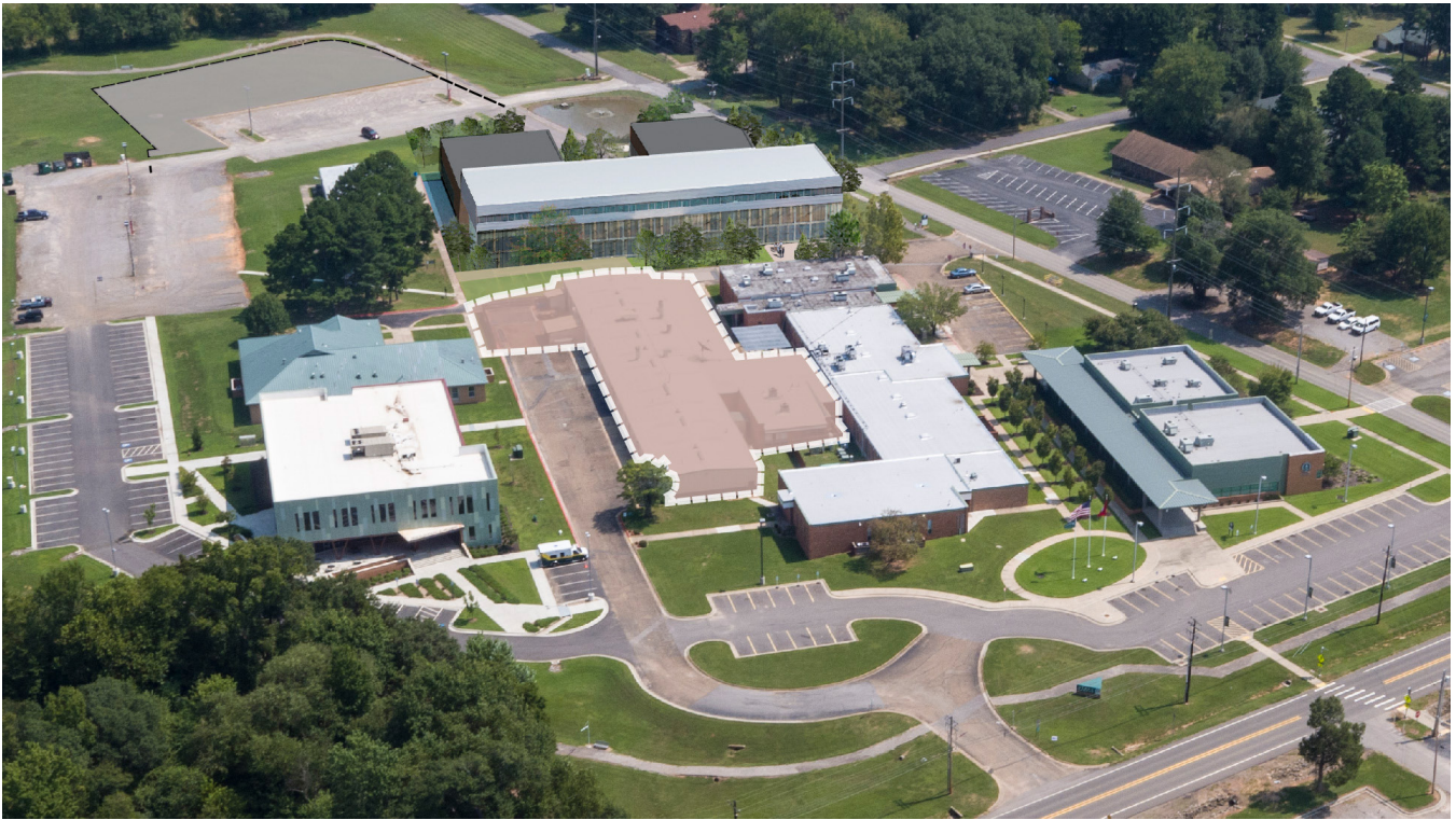
Ozark Campus aerial highlighting the removal of the Shop Building.
